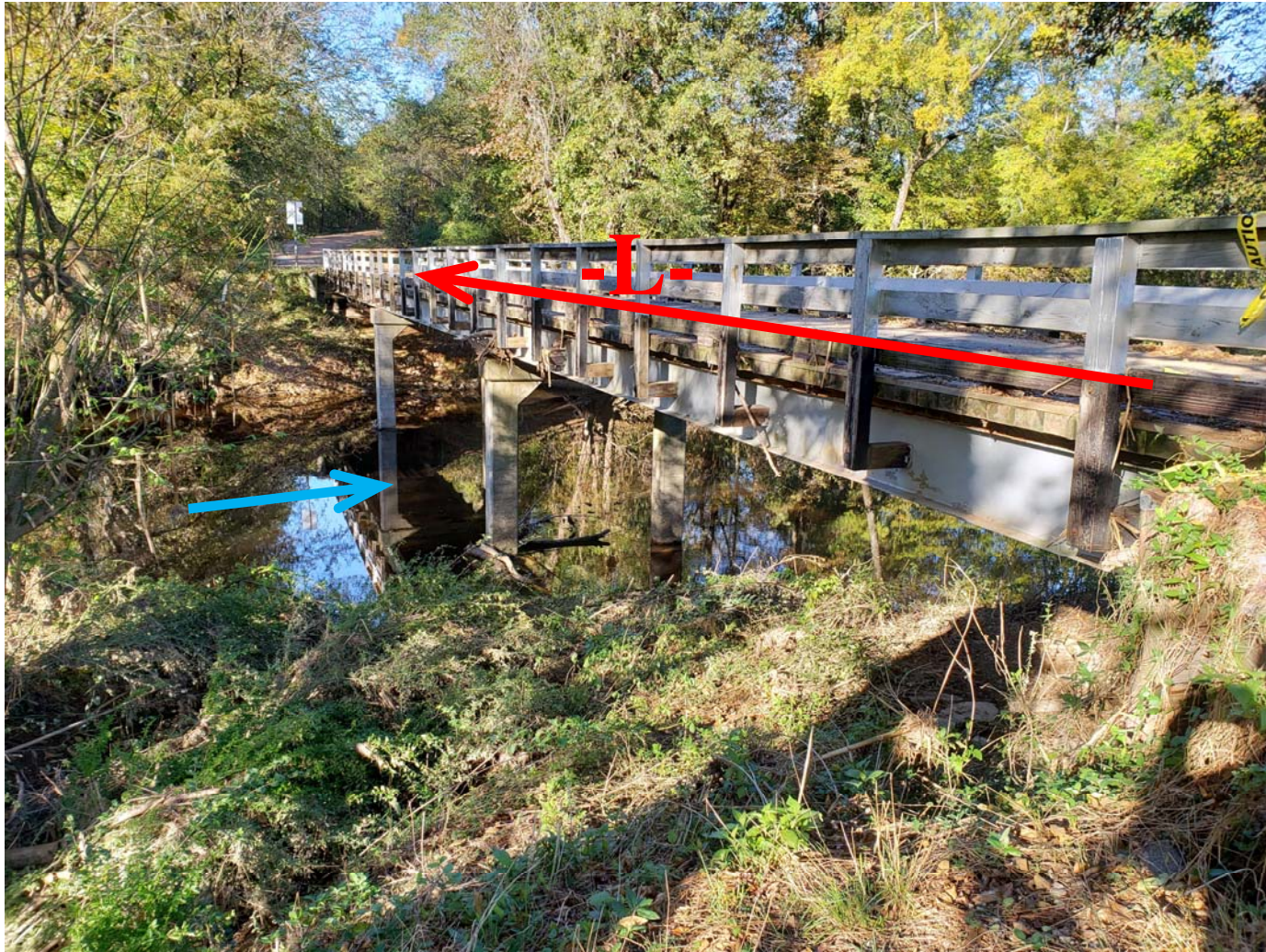
Looking West Towards End Bent 1
